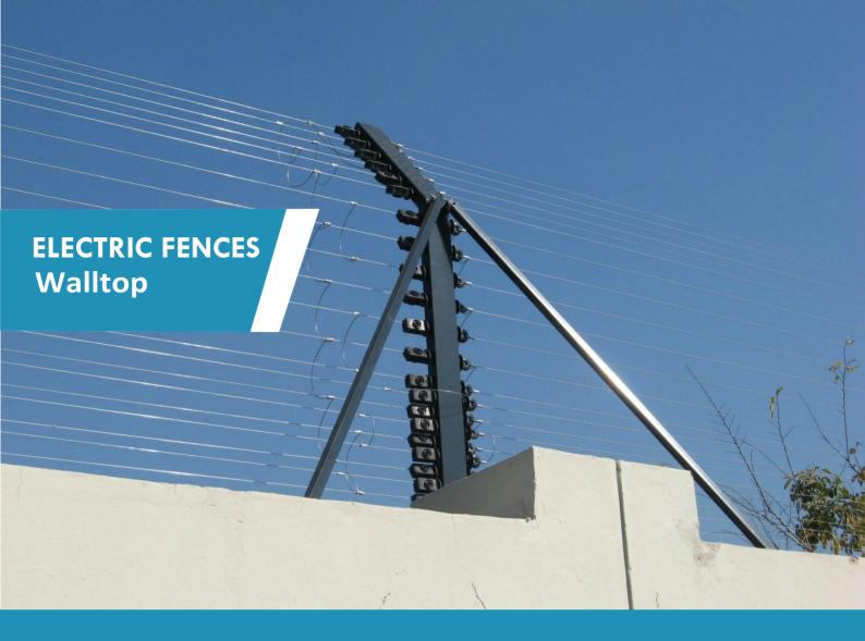
Wall Top Electric Fencing: A wall-top electric fence normally consists of 3m spaced steel brackets made from flat bar or square tube attached to a wall, supporting 5 to 10 vertical alternate live and earth electric fence wires.
