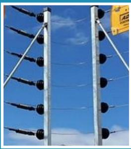
Free Standing Electric Fence: A free standing Electric fence is a permanent self-standing electric fence. The fences are predominantly for security purposes, are normally 1.8-3m in height with alternate live earth 2.24 High Strain Line Wires spaced 10cm apart.
